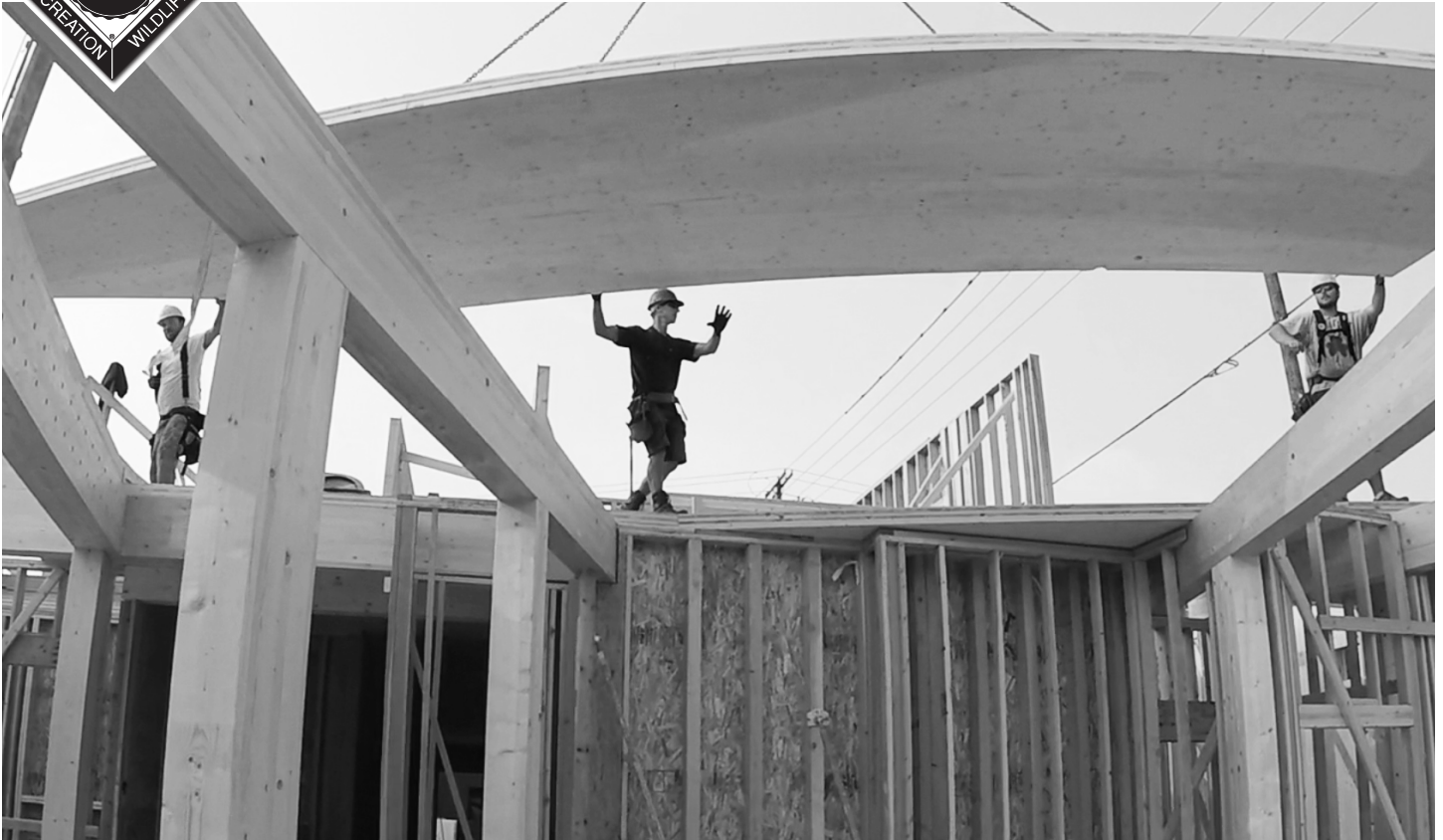
The Lark Hotel used cross-laminated timber extensively in its recent expansion. Photo by: Think Tank Design Group, Inc. Bozeman, MT.
