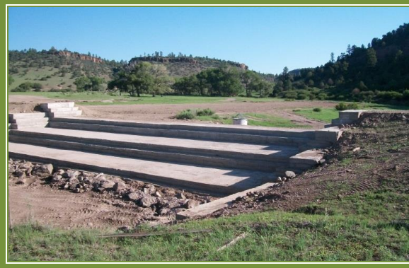
Structure # 2 - installed in 2012; first major flood flow in 2013; it will raise the creek level 10.5 feet.
