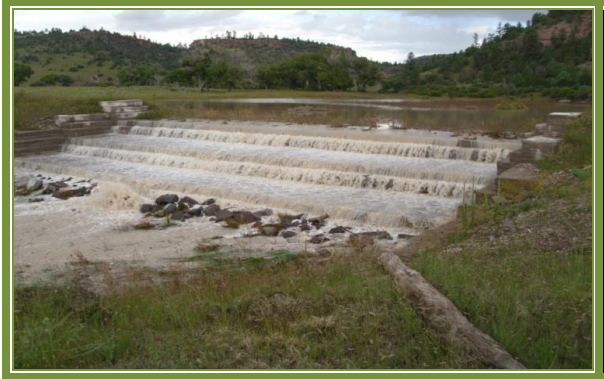
Structure # 2 - installed in 2012; first major flood flow in 2013; it will raise the creek level 10.5 feet.
