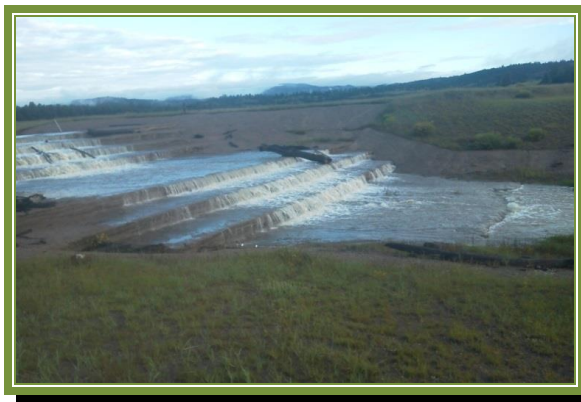
Structure # 1 - has been in place since 2000; it has raised the upstream creek level 10 feet so far.
