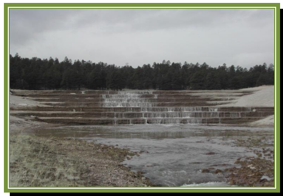
Structure # 1 - has been in place since 2000; it has raised the upstream creek level 10 feet so far.
