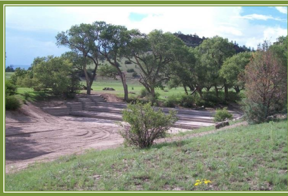
Structure # 3 - installed in 2012; first major flow in 2013; it will raise the creek level 10 feet.
