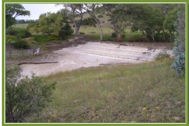
Structure # 3 - installed in 2012; first major flow in 2013; it will raise the creek level 10 feet.
