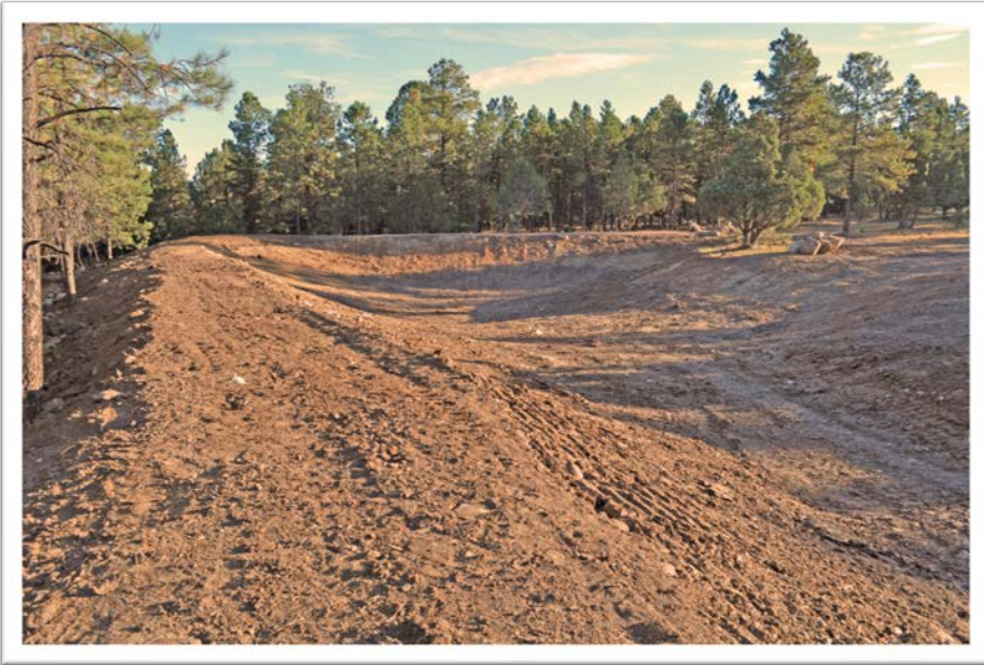
Finished pond ready for the rain! Note the top and backsides of the embankment are covered with the reserved top soil. (2010 Photo by J. Riddick)
