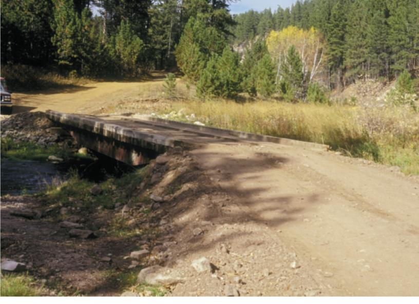
Compact fill material to prevent seepage and failure. Armor the inlet and/or outlet with rock or other suitable materials.
