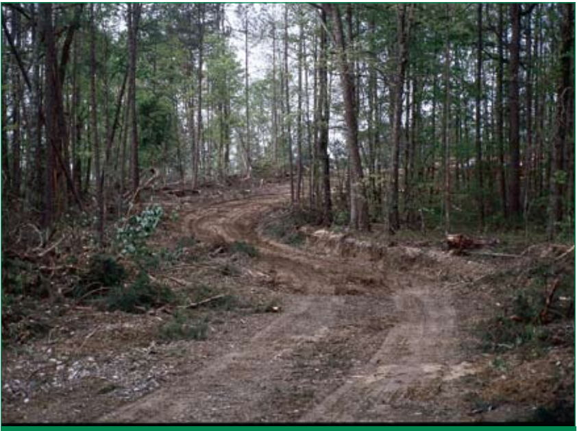
Temporary Active Road
