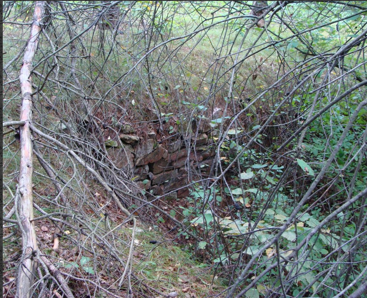
stone foundation wall and depression
