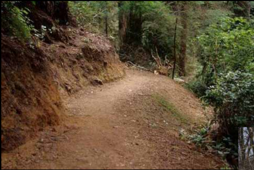
New trail with steep backslope
