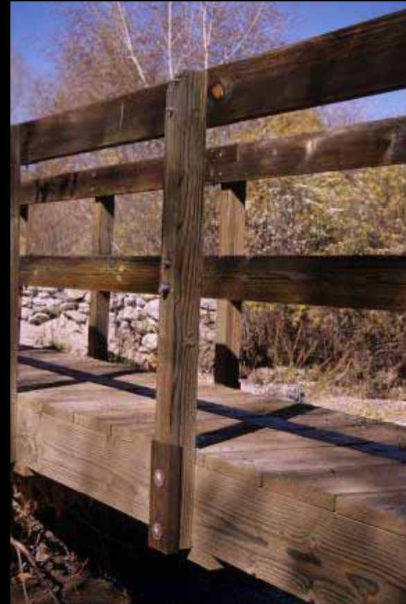
Attached to Girder
