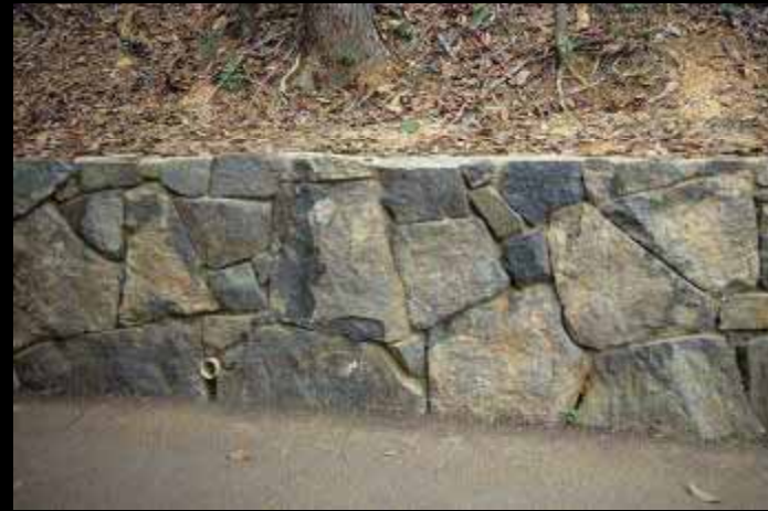
Fitted, Mortared Rock
