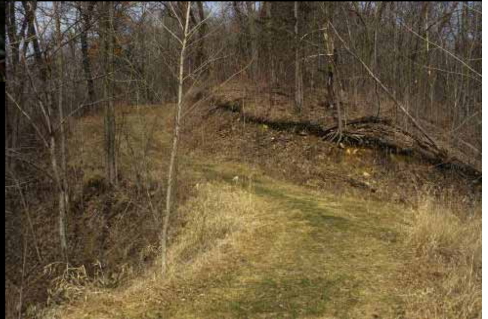
Old trail with eroding backslope
