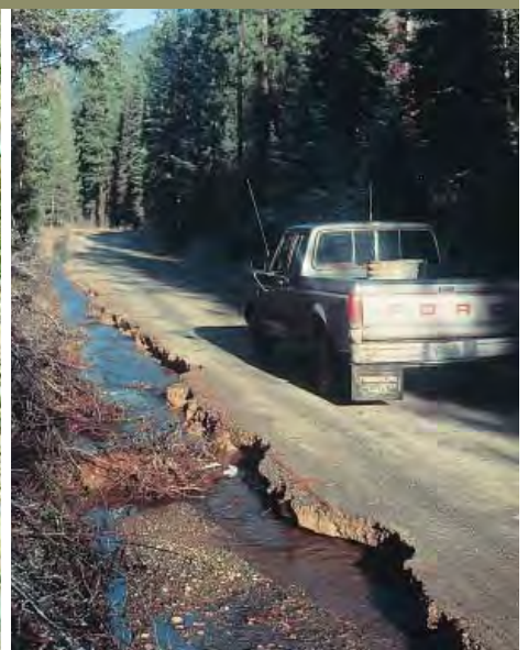
This plugged crossdrain culvert and washed-out catch basin can be a source of sediment.
