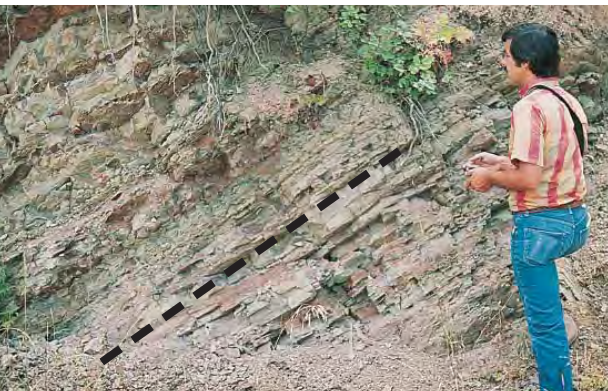
Rock layers that slant with, rather than into, the slope are a clue to potentially unstable bedrock conditions.
