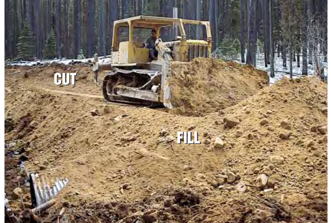
Cut-and-fill road construction is common for gentle terrain.
