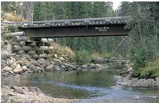
Bridges are best for large streams and those plagued with floatable debris problems. Bridges and arches have the least impact on fish.
