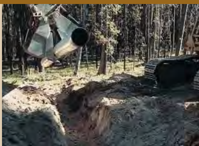
Seat the culvert on the natural slope. Bedding material should be free of rock or debris that might puncture the pipe or carry water around the culvert.
