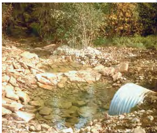
Step pools at culvert outlets can sometimes correct the problem of hanging culverts by allowing fish to rest before attempting passage.
