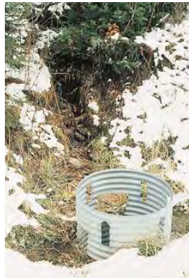
Drop inlet installed at a ditch relief culvert inlet slows water, helps settle out sediment and protects the culvert from plugging.
