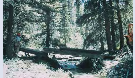
A portable railroad flatcar provides access across streams with minimal disturbance to streambanks or bed. Select locations with firm soil banks, level grade and minimal vegetation clearing.
