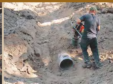
Compact soil at least halfway to prevent water seepage around sides. Be sure outlet extends beyond any fill and empties onto an apron of rock, gravel, brush or logs.
