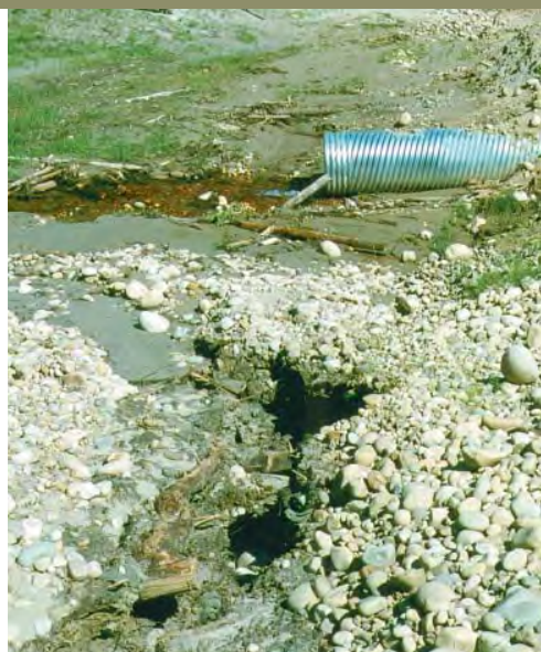
Water runoff formed these long narrow chutes or rills, running downslope on the surface of this road cut slope. It is a source of sediment.
