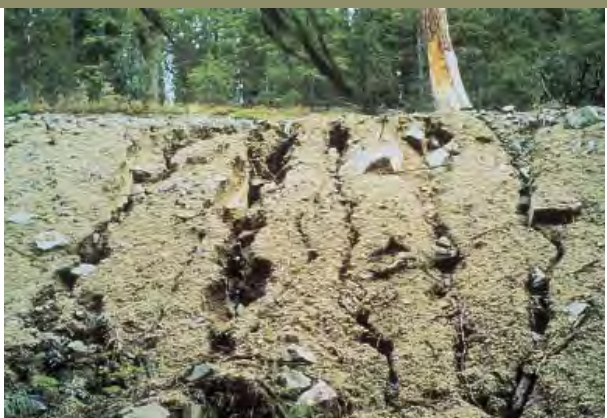
Water runoff formed these long narrow chutes or rills, running downslope on the surface of this road cut slope. It is a source of sediment.
