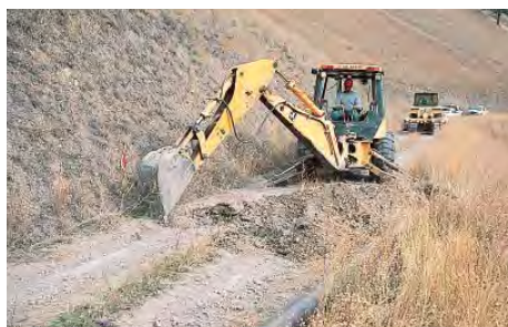
A backhoe is the best choice for open top pipe culvert installation.
