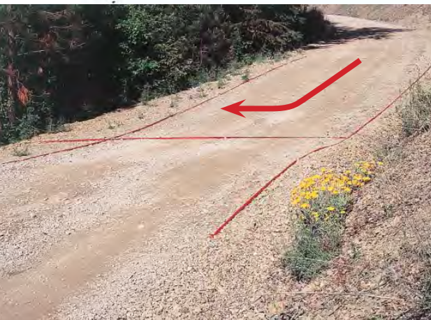
Use at least 50 feet for approach and runout. More on steeper road grades.
