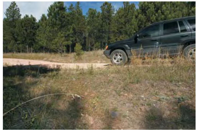
The drain dip bottom is sloped to carry water from inside to outside of road surface, onto natural ground.
