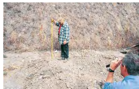
Pipe bed must have a grade of 8%.
