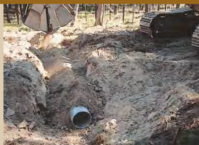
Cover with soil, using at least one foot or one-third the culvert diameter, whichever is greater. Avoid punctures from large rocks.
