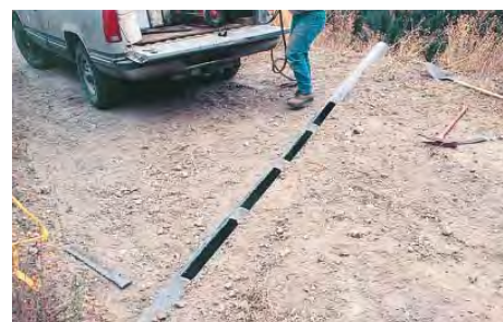
Slots are wide enough for cleaning but do not damage tires.
