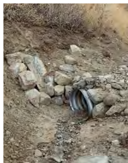
Rock-armored catch basins prevent water from eroding and undercutting the culvert inlet and flowing under the culvert.
