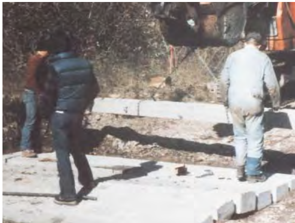
Concrete planks, fastened together and stretched across the streambed, provide an "improved" ford crossing.
