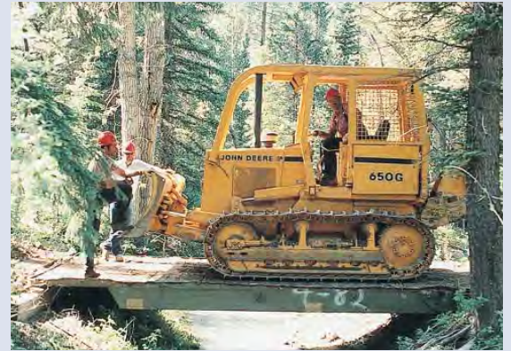
A portable railroad flatcar provides access across streams with minimal disturbance to streambanks or bed. Select locations with firm soil banks, level grade and minimal vegetation clearing.
