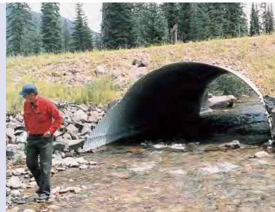
Bottomless arches leave the streambed intact, making it easier for fish to pass. Natural streambed roughness creates pockets of low water velocity where fish can move comfortably. Bedrock or concrete footings are required.
