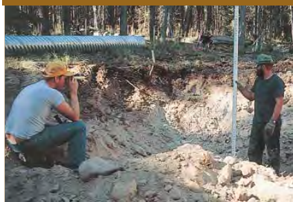
Ensure proper tilt of culvert. At least five inches in every ten feet.
