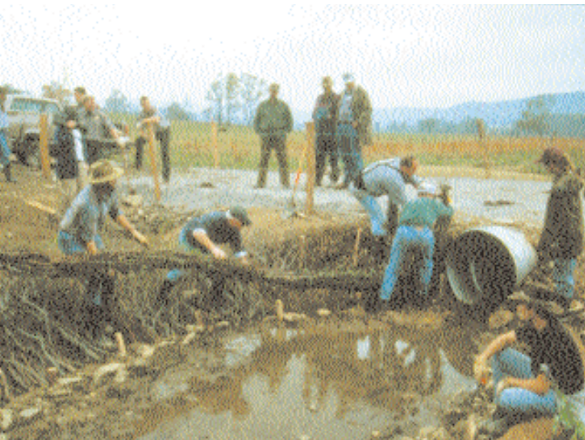
Installing a large culvert can improve fish passage.
