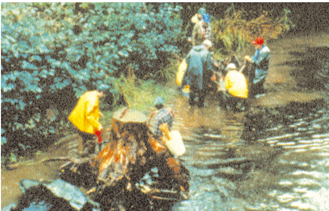
Rootwads placed in stream to protect bank and provide cover.
